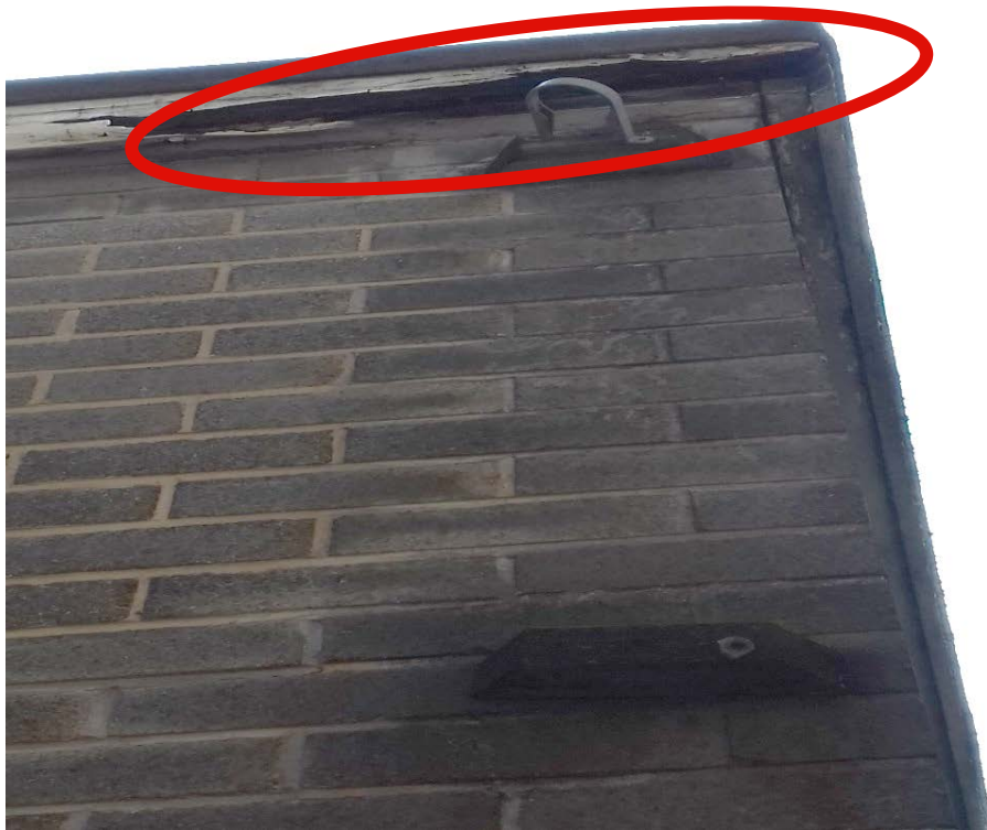
Photo 3- Building 2, Development Parcel F
